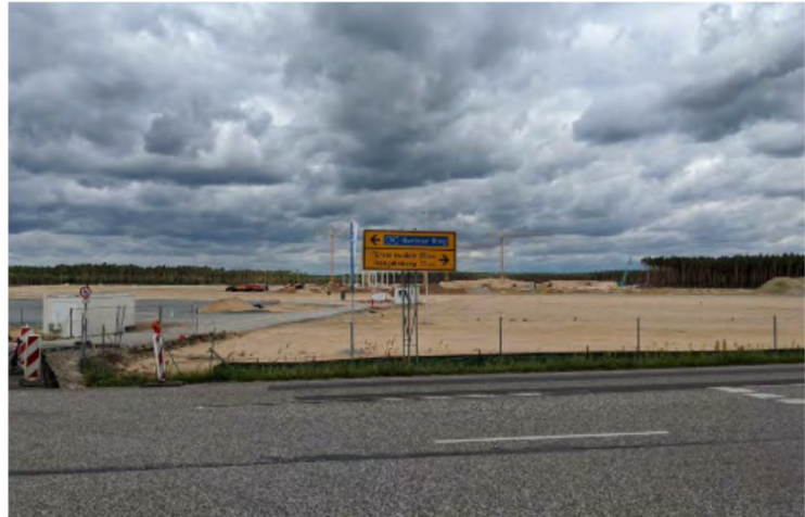
The Gigafactory’s southern entrance under construction in July.
